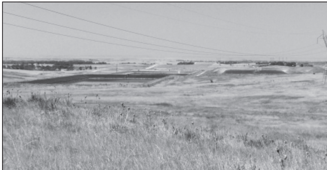
Evaporation ponds at the Crow Butte in situ leach uranium mine near Crawford, Nebraska.
